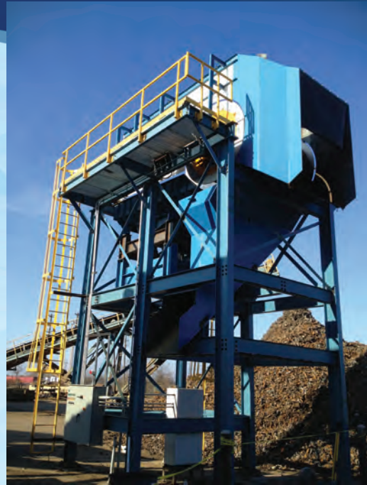
BPS custom engineers platforms and structures based on our customers' needs.
